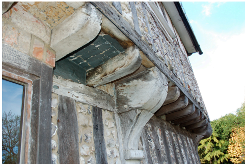
Fig 26 Jettying of first floor of Tudor House
