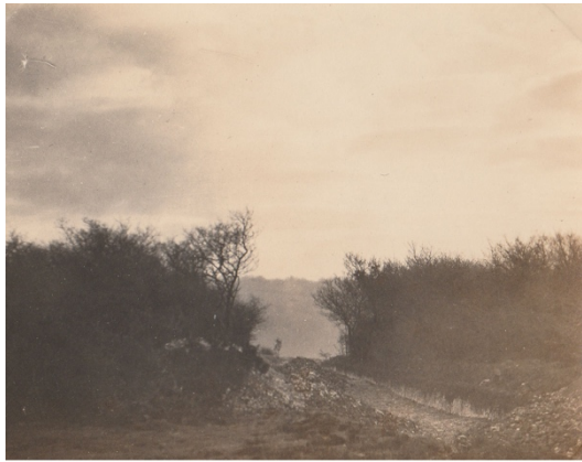
Cutting out the new road March 1922
