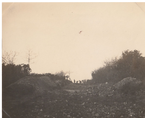
Cutting out the New Road March 1922
