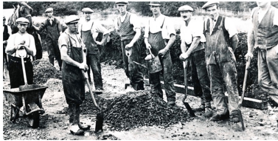
Fig 8. Groundsmen preparing asphalt for the driveways
